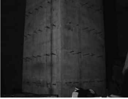
Figure 3. A view of concrete pillar in Fetr6 underground mine (Faryab Co. 2008).
