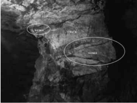
Figure 6. Condition of Pillar No.19 in phase 1 of Fetr6 underground mine (Faryab Co. 2008).
