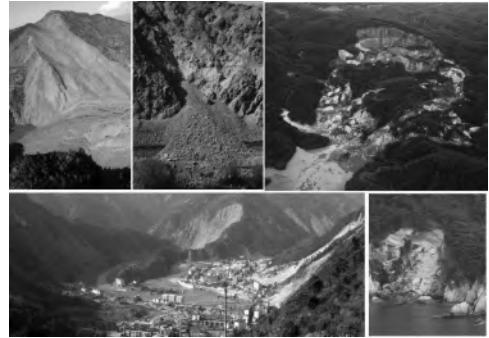
Figure 40. Examples of slope failures induced by earthquakes.
