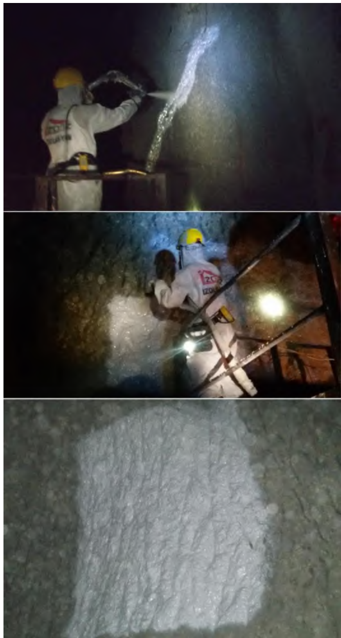
Figure 5. TSL spraying on face
