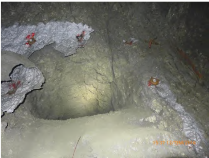
Figure 6. The face after blasting
