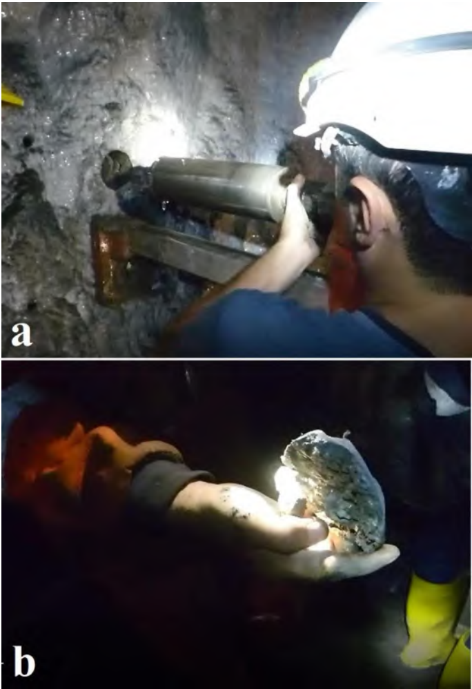
Figure 9. a) Core sampling on the TSL applied face, b) cored TSL
