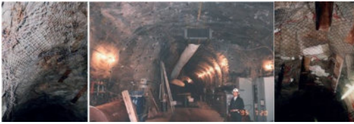
Figure 2. Rockburst and spalling of underground openings in hard rock mass
