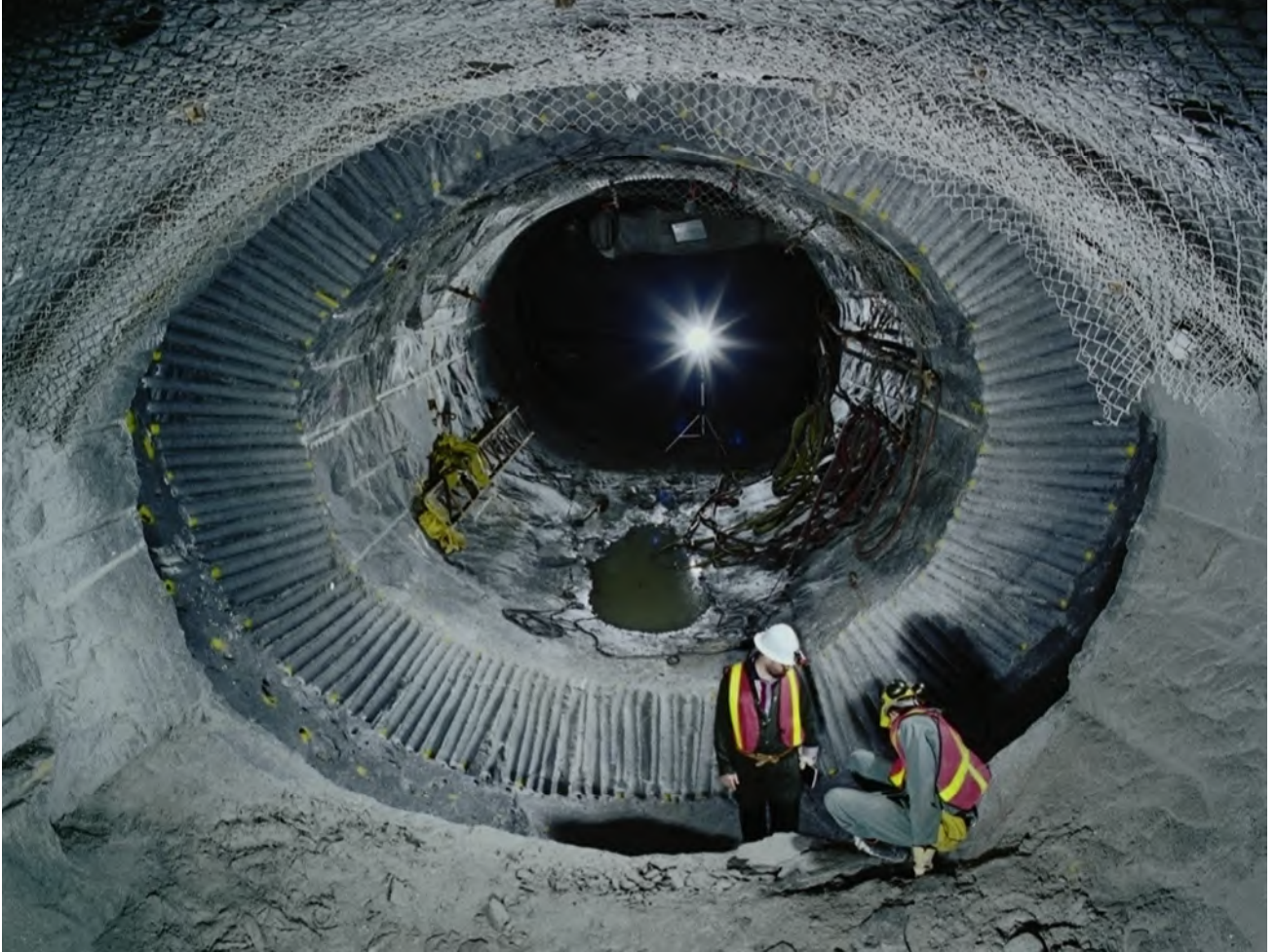
Figure 7: Elliptical tunnel. Note no rock failure around the perimeter (Picture from The Underground Research Laboratory, Pinawa, Manitoba, Canada).
